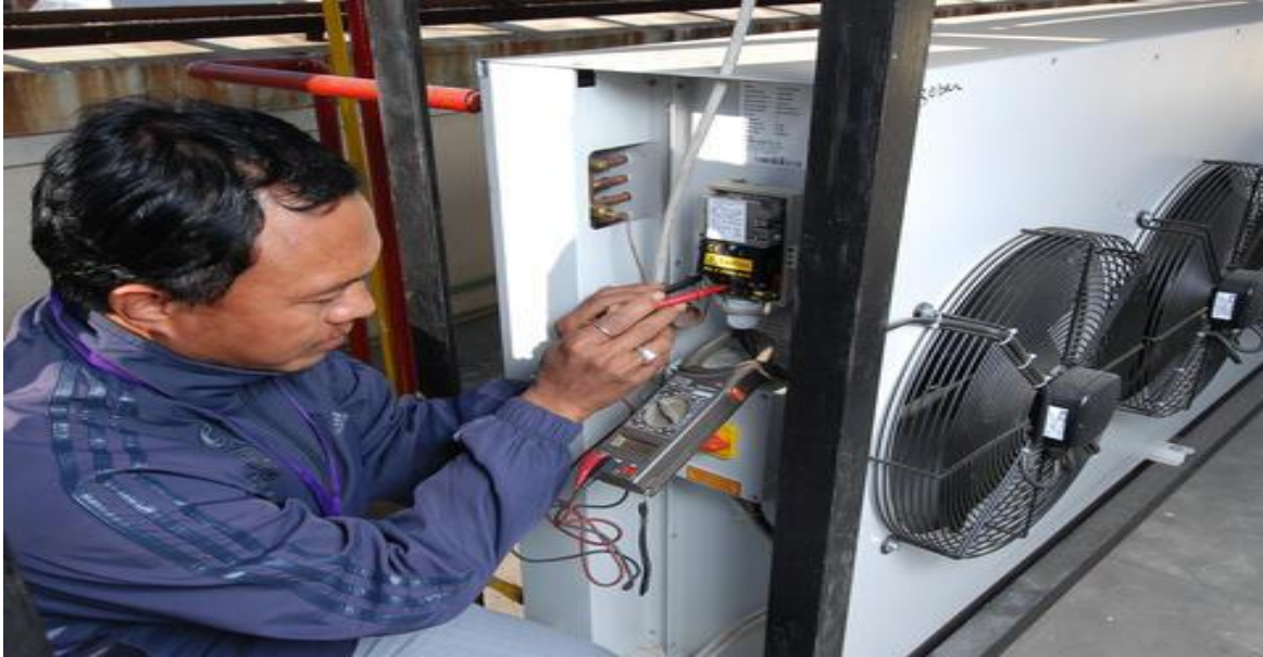
Figure 6: Dismantling of refrigerator
